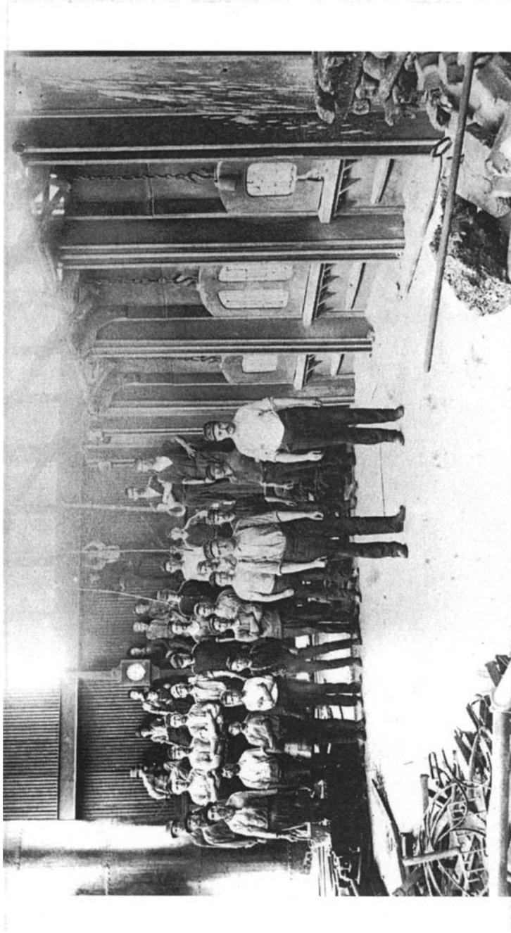
Figure 4. **Open Hearth Furnace #1.** Open hearth technology was dependent on invisible chemical reactions that changed according to the contents of the pig iron, scrap, fuel, and chemicals they used, along with the temperature of the fire, the length of the heat, and the size, shape, and condition of the mold it was poured into.
