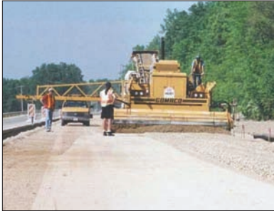
Trimming a granular subbase
