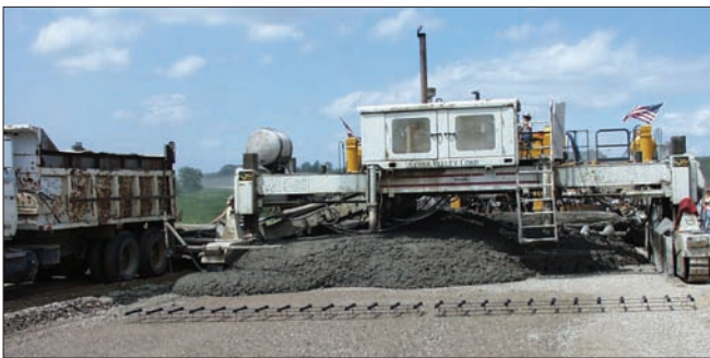
Top to bottom: ready-mix truck, dump truck with agitator paddle, mixture in front of paver
