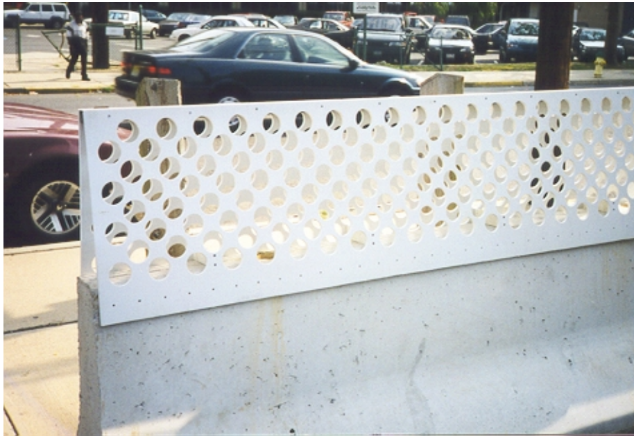
Figure 5. Prototype of side-mount CGSPF using recycled plastics (Opening can be any shape or circular as shown; H = 24-inch, %void = 41%, Weigh = 5.3 lb/ft)
