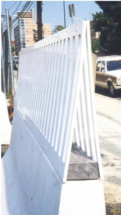
Figure 6. Prototype of top-mount CGSPF using recycled plastics
