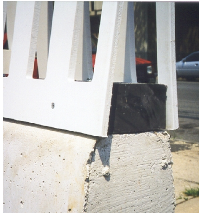
Figure 6. Prototype of top-mount CGSPF using recycled plastics
