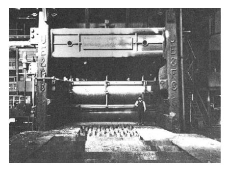
Figure 2. **204-inch Four-high Reversing Mill.** This size of this mill dwarfed the 84-inch mill built in 1870 (Chap. 4, Figure 2). It was capable of rolling steel 25 inches thick and 16 feet wide.
