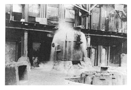
Figure 2. **Tapping an Open Hearth Furnace.** The molds for filling are in a pit near the furnace so that the steel can be poured directly into them.
