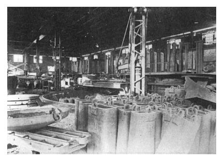
Figure 3. **Open Hearth Furnaces, Ingot Molds, the Soaking Pit and Crane.** Lukens built open hearths in sets—Open Hearth #1 (1890) had two furnaces, Open Hearth #2 (1899) had four furnaces, and Open Hearth #3 (1918) had eight furnaces.
