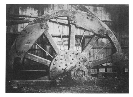
Figure 3. **Flywheel for Power.** This flywheel was connected to the waterwheel to stabilize the vibrations and add more power in the 1850s.
