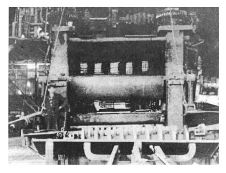
Figure 2. **84-inch Steam Powered Mill.** This mill, built in 1870, was the first significant expansion that Lukens made. It was later dwarfed by the 204-inch mill opened in 1918 (Chap. 6, Figure 2).
