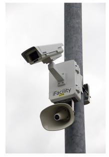
CCTV camera and iFacility IP Audio speaker on a pole by RickySpanish used under CC-BY-SA 4.0
