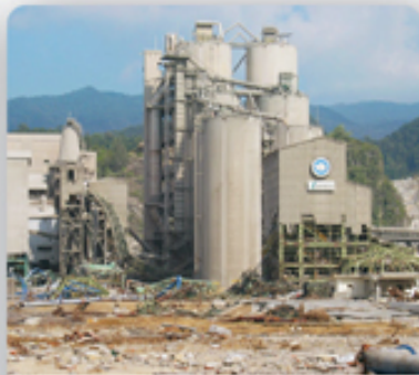
Cement factory damaged by tsunami.
