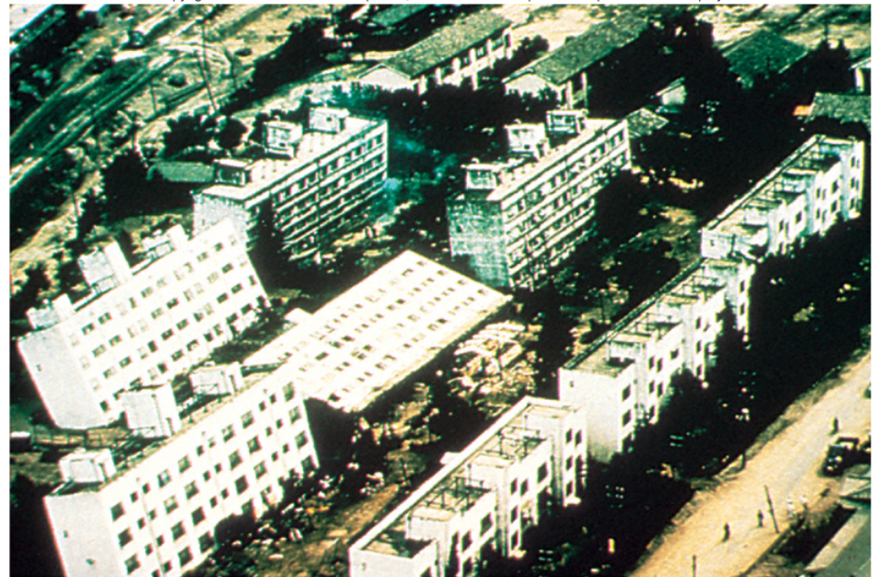
b. Apartment buildings collapsed due to liquefaction after 1964 Niigata (Japan) earthquake.
