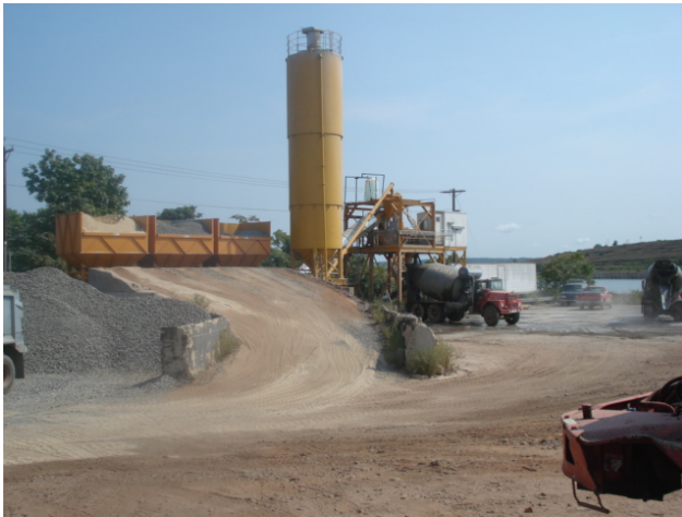
Because V. Paulius plans to produce over 54,000 CY of concrete for their two Carteret projects, they installed their own plant on-site.
