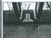
Ledger board and joists in place using the Simpson Hanger
