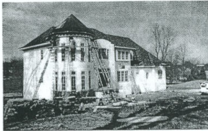
COMPLETE ICF BUILT SHOW HOME IN VIRGINIA; COMPLETE WITH RADIUS WALLS, OVAL/CIRCLE OPENINGS; STONE, BRICK, STUCCO EXTERIORS - SHE'S A BEAUTY - FEAR NO DESIGN!
