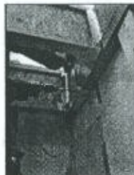
Ledger board and joists in place using the Simpson Hanger
