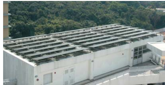
Figure 13-10 Three bays of Canopy system to suit the standard HK School Planning Grid.
