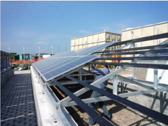
Figure 11-10 PV panel installation
