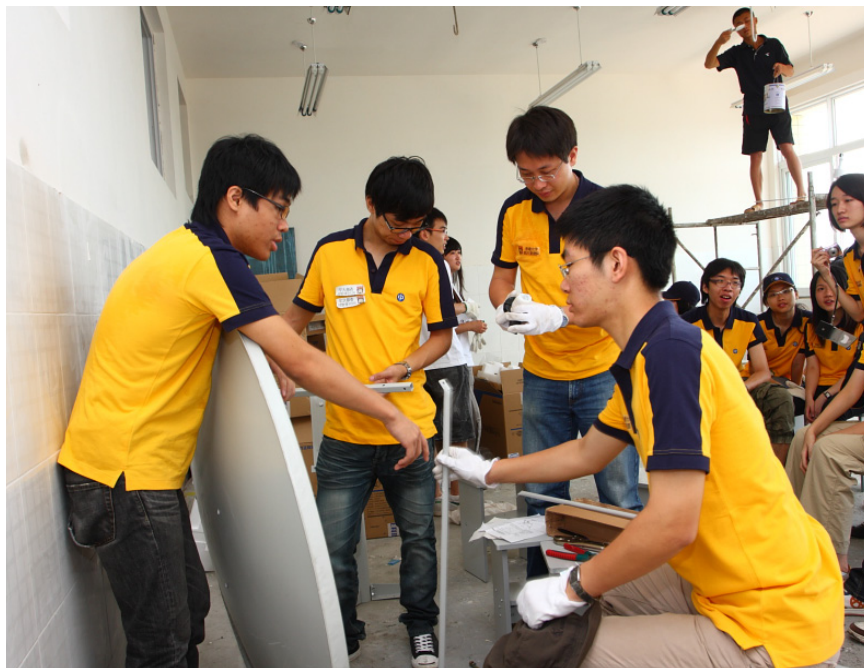
Students are installing the satellite
